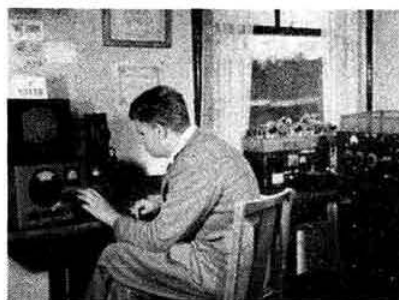
G3FXB, who came fifth with 3,510 points, operating his station in Southwick, Sussex. The receiver is a Hallicrafters SX24 with a modified RF26 unit as a converter for 10, 15 and 20m. The transmitter, using push-pull 807s, is in the rack at the extreme right of the picture.
